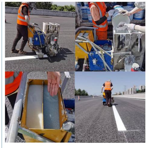
HG-20MM-II is to put two kinds of coatings in the same barrel separated. After discharging the coatings from the tank, the coatings are fully stirred by an electric stirring shaft. After mixing in the crossing hopper, the chemical reaction is carried out. Finally, the marking is done through the crossing hopper. Compared with spraying two-component marking, scraping marking has the advantages of thicker marking thickness, longer wear resistance, better reflectivity and more uniform mixing.
