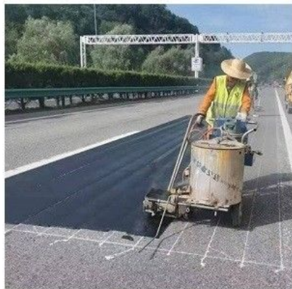
reticular crack
